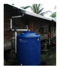
Figure 6: The main component rainwater harvesting system
